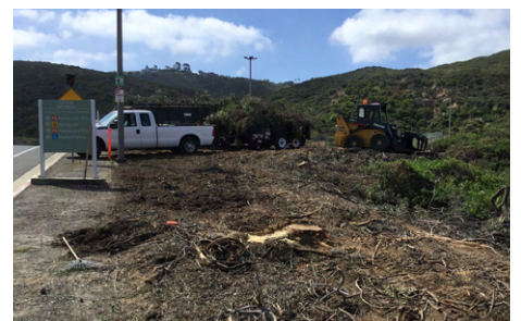
PALM CANYON RENOVATION
