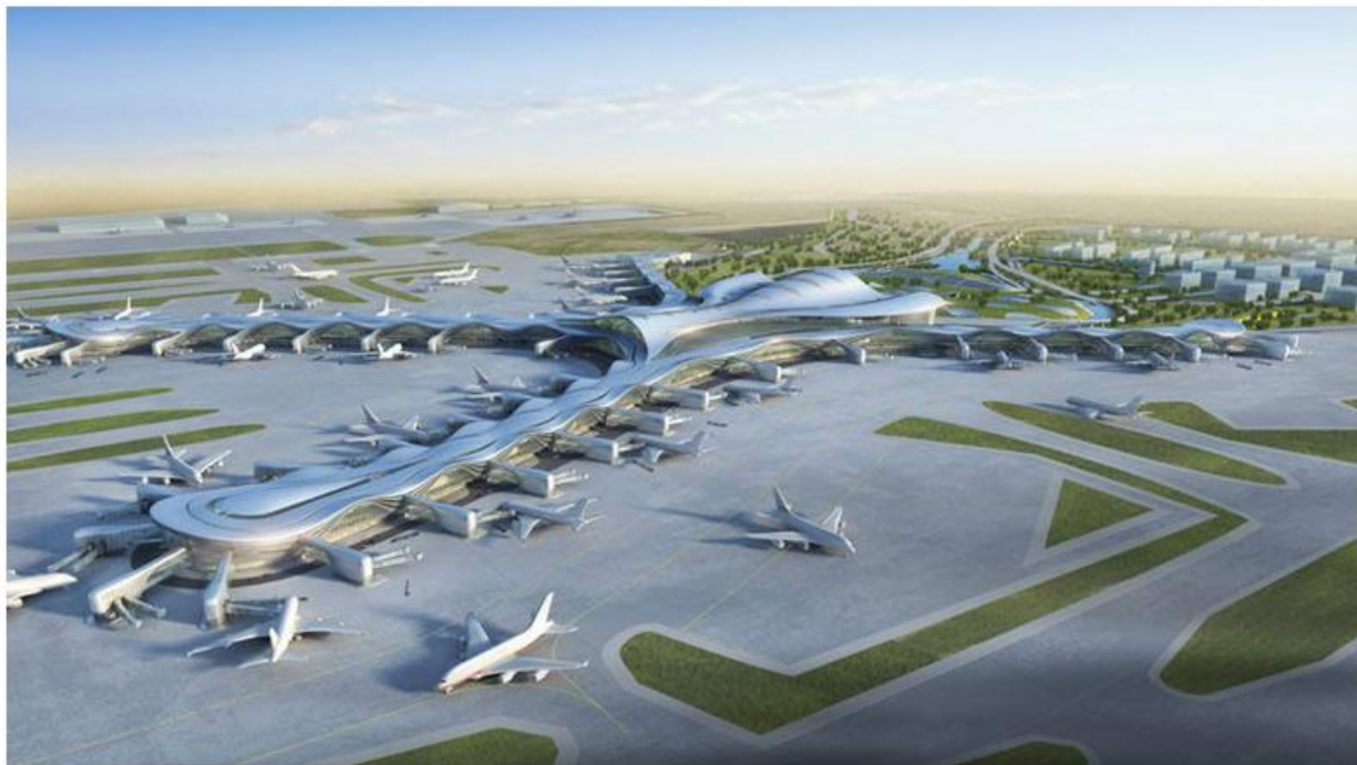
Figure 4: Abu Dhabi International Airport Midfield Terminal Complex
