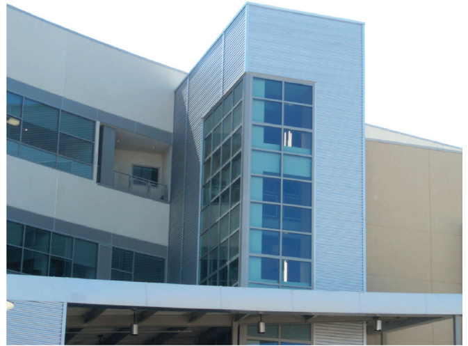
Markstein Hall, home to the College of Business Administration and other programs.
